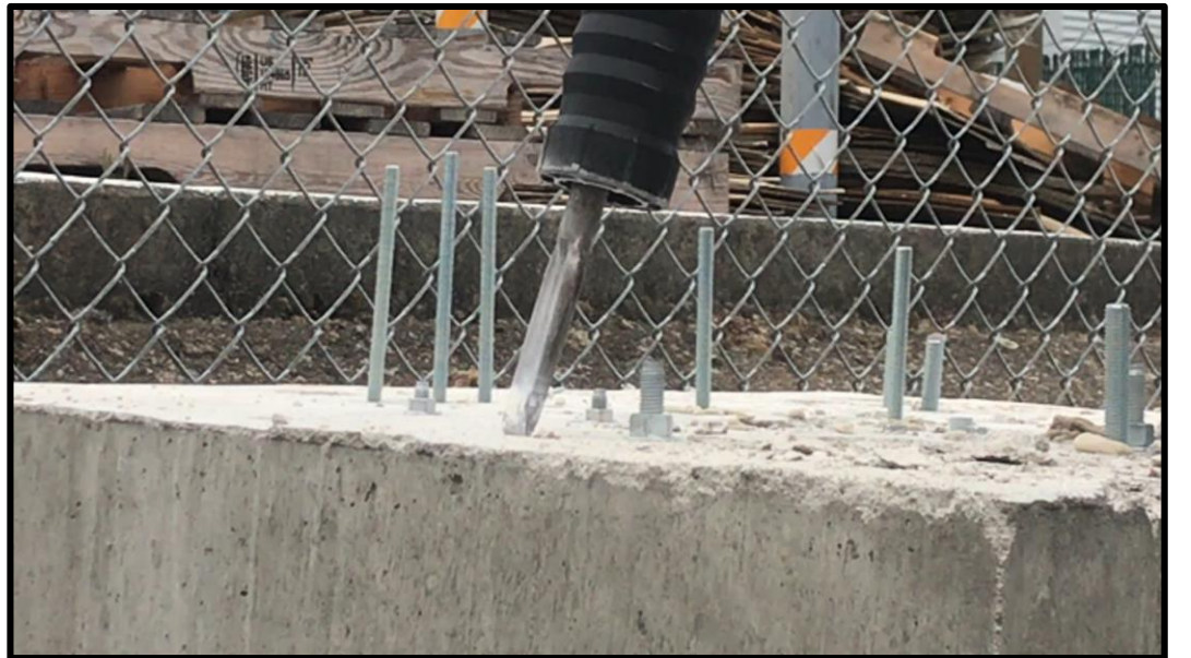
Figure 2: Jackhammer with vacuum on
