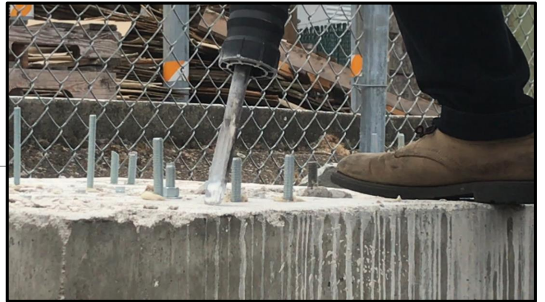
Figure 1: Jackhammer with vacuum off
