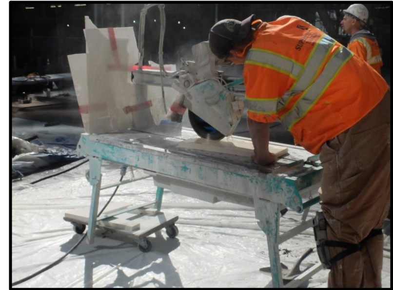
Worker wet-cutting a piece of stone
