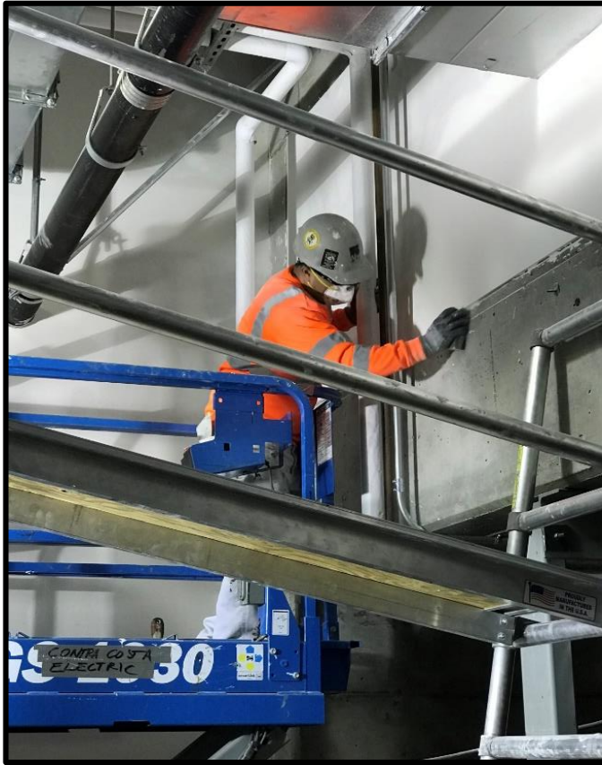
Laborer sanding drywall wearing a respirator
